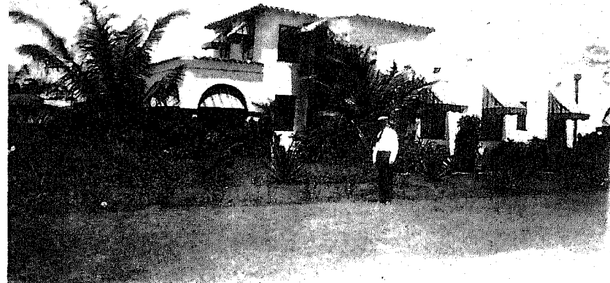
801 Hibiscus Street, taken about 1935 from Paloma Avenue looking west. Originally the Aiken home, Fred Aiken is standing in the road.
