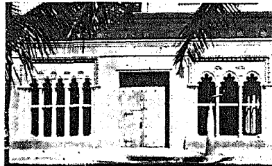
Royal Palm Way Building Mizner Cast Stone was used in the building shown above. Note the varied style and texture.
