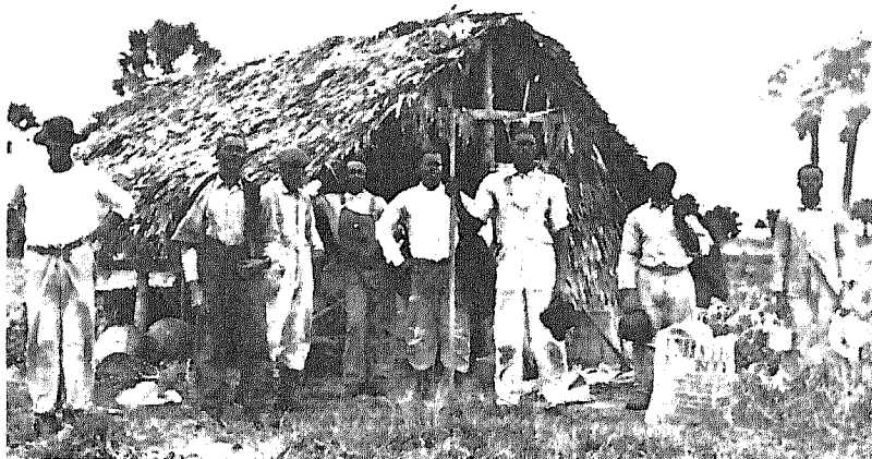
Farm workers at Chesebro Pineapple fields. Sheds were wood frame, covered with palmetto fronds. Names of men are unknown.
