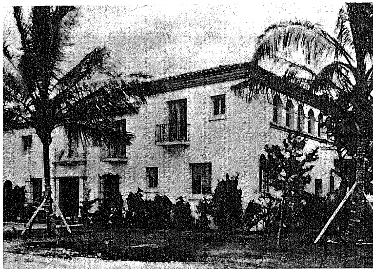
The North Building, northern facade on Camino Real, 1926. Photograph: Pacific Coast Architect, R. Reynolds Clark.
