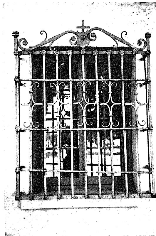
The North Building, window grill. Photograph: Fred Eckel
