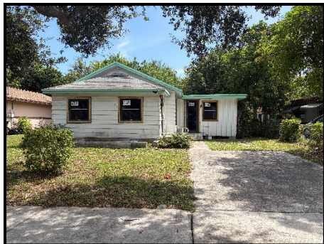
Fountain House at 156 NE Pearl Street
