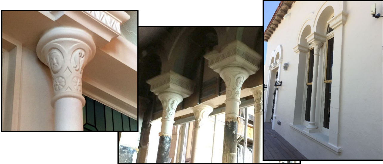
Mizner designed columns visible inside and outside the Palm Court
