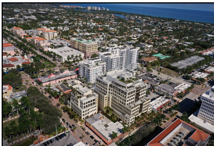
Aletto Square office complex being built at Palmetto Park Road/ Boca Raton Road.
