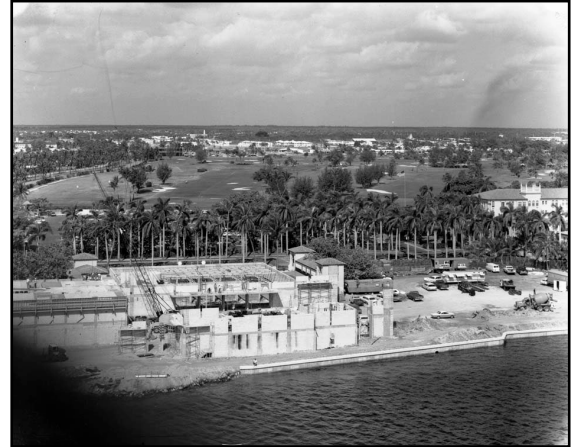
The Garden Pool, left, and the Great Hall construction at right. The Great Hall incorporated the pool walls into the building and the old pool itself was replaced with a large meeting room.
